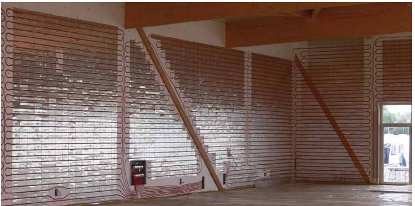
Presentation of wall heating with dry construction system
